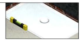
8. Bed down the Flowaway wet floor base using a suitable material which will fill out any voids. We recommend the use of a weak sand and cement mix, thistle plaster or tiling adhesive ensuring all areas are supported and level.
