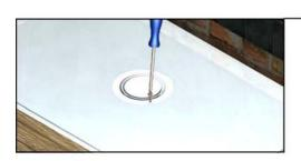
17. Secure the waste gully trap in place using screws.
