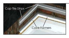
12. Following the manufacturer's instructions, mount a cove former and cap tile strip to each of the 4 walls using the appropriate adhesives respectively.
