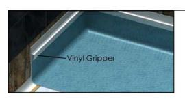
13. The vinyl flooring should be laid throughout the room, covering the Flowaway® and cove formers, and inserted into the vinyl gripper of the cap tile strips around the perimeter of the room.
